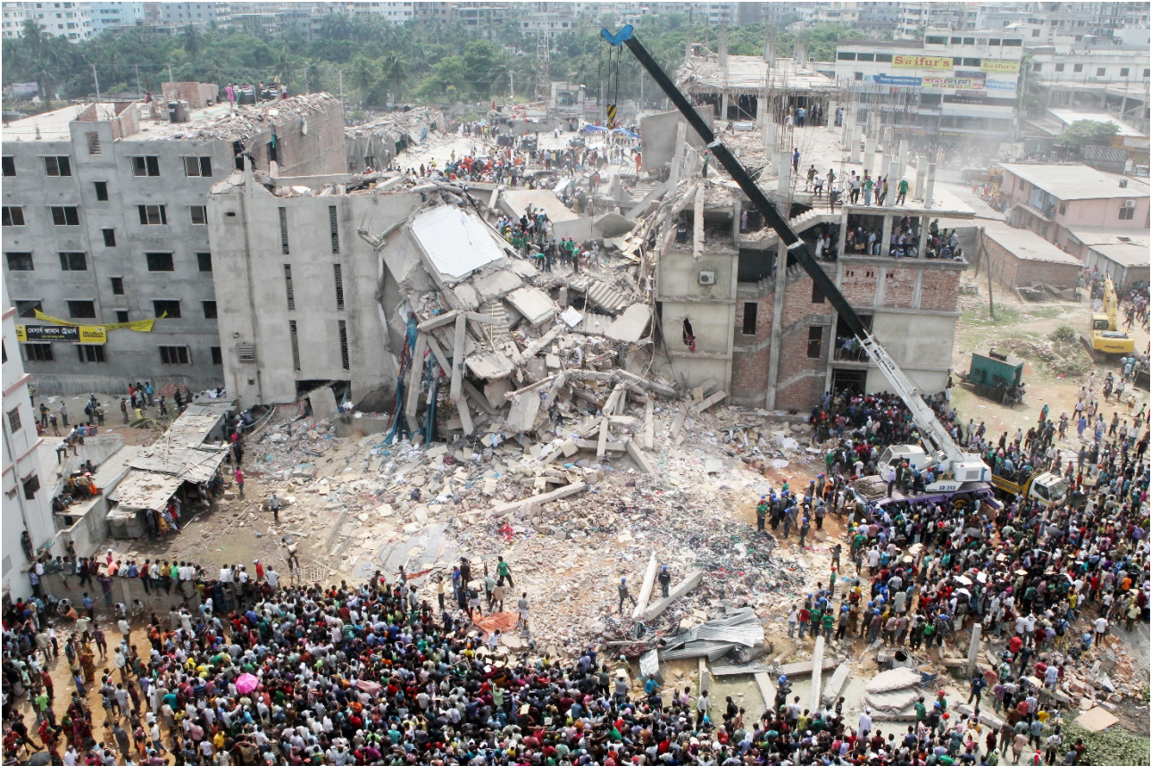
Rana Plaza after its collapse in April 2013
